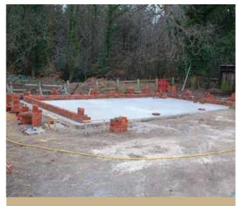
Having set out, the concrete has been poured and the brick plinth is in progress (typically three courses).
