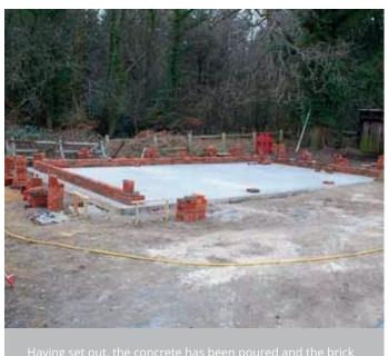
Having set out, the concrete has been poured and the brick plinth is in progress (typically three courses).
